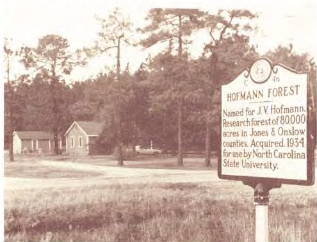
Hofmann Forest Headquarters Buildings
